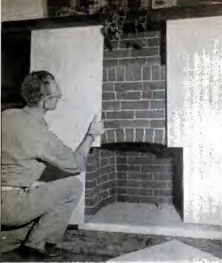
Above, each section of the front panel should be tried to make certain of the fit for best results
